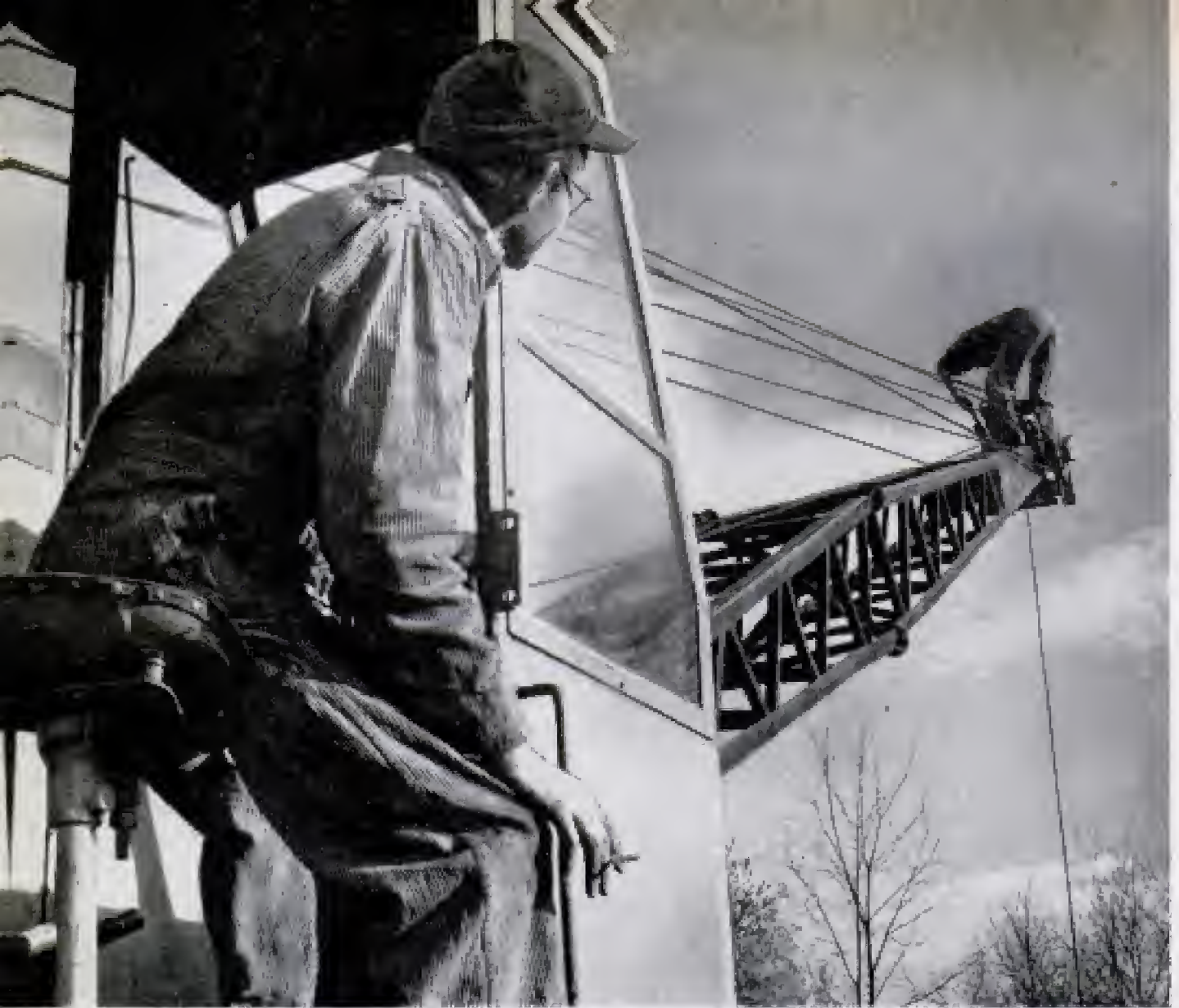
Five dump trucks stood idle until Hamlin climbed out on the end of this crane to unsnarl jammed cables
